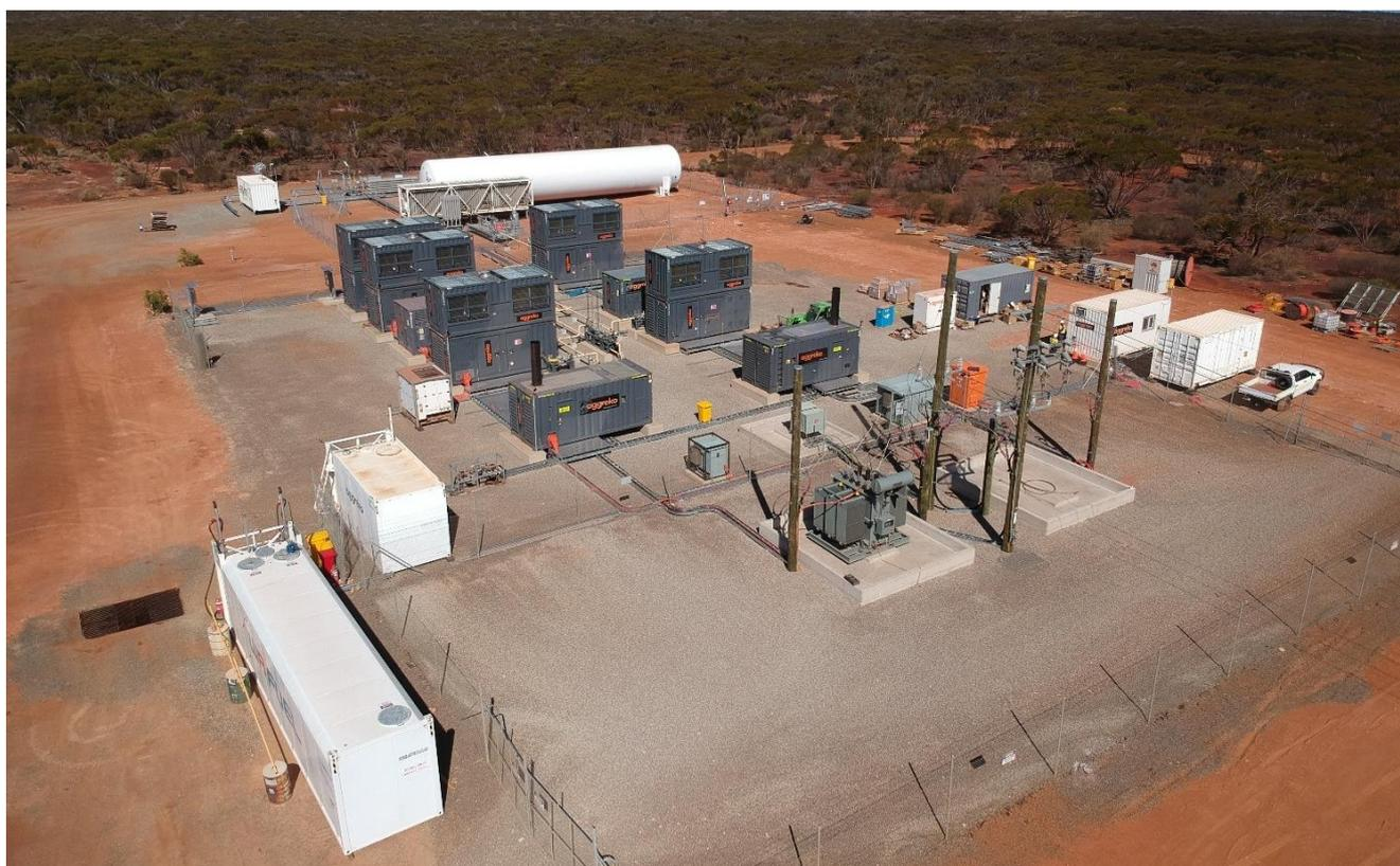
*Figure 4: New Power Station with LNG facility in background pre-commissioned*
